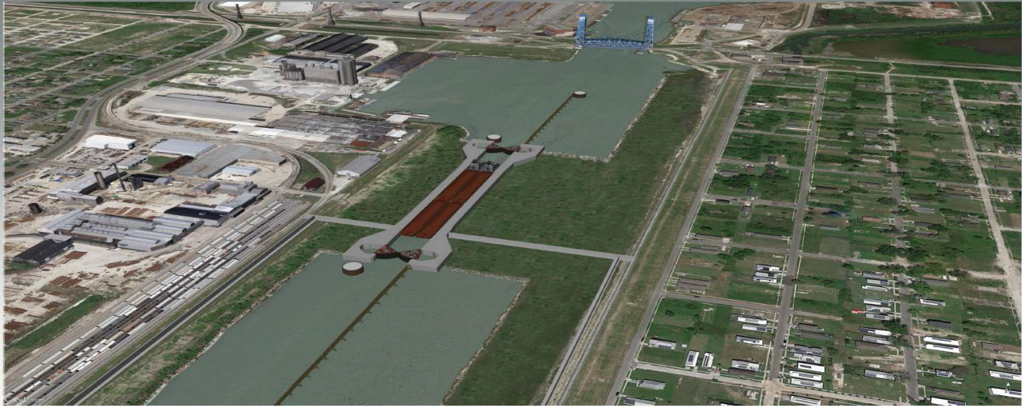
New 900 feet long by 110 feet wide IHNC Lock, with a sill elevation of -22.0 feet NAVD88.
