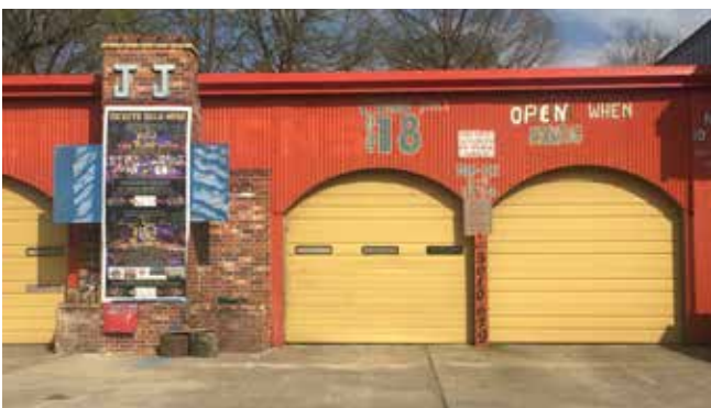
J & J's Inspection 6710
